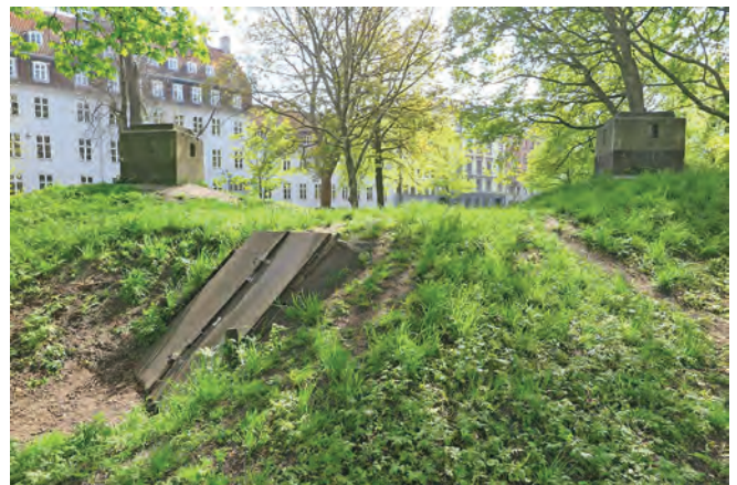
Cold War civilian shelters grouped around Copenhagen Castle moat
